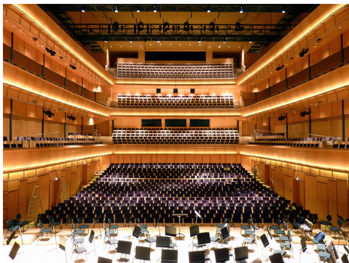
Figure 5: Fartein Valen Concert Hall, Stavanger, Norway. The side balconies are free from the side walls and have “downstands” integrated to provide downkicking early reflections. The balcony form is similar to reflector types D and E studied here in 2D BEM.
