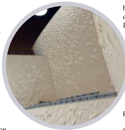
Top: The symphony hall has two levels of convexly curved and inclined walls designed to create early lateral and enveloping reflections
